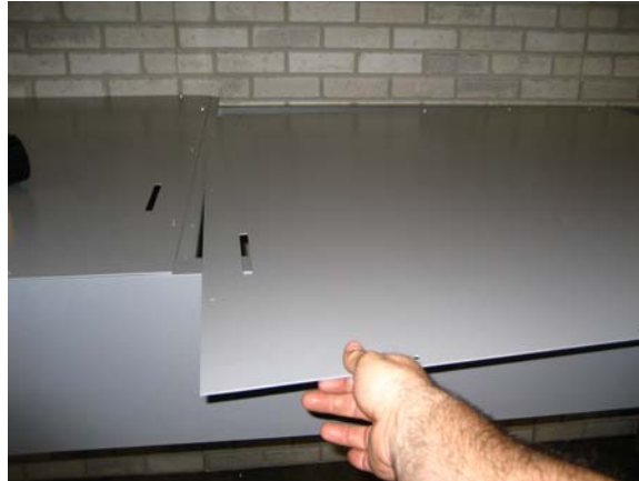
Insert slot covers as shown and attach using 10-32 hex nuts provided
