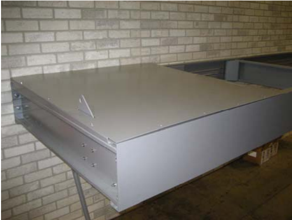
Slip panel over beginning of section
